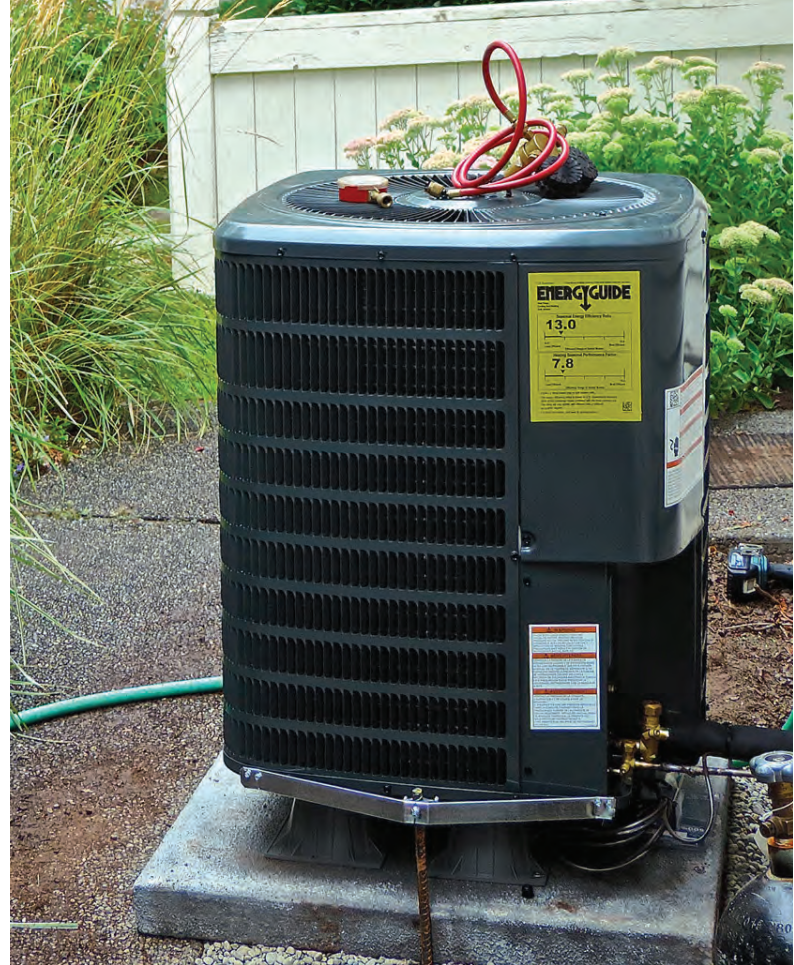
An air-source heat pump compressor outside the home can distribute hot and cold air through your existing duct system.
