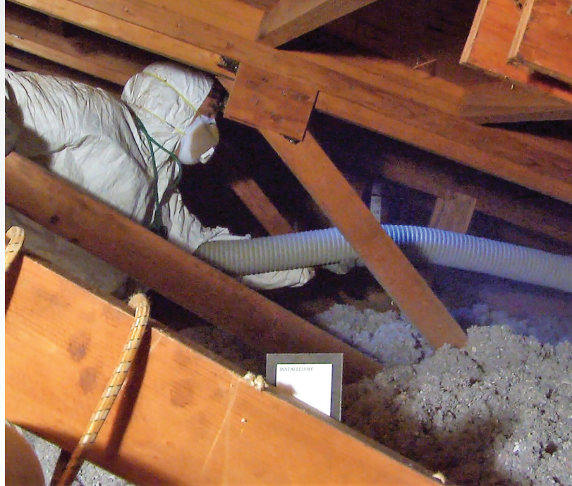
A contractor installs blown cellulose insulation in an attic to minimize energy waste. PHOTO COURTESY OF PROJECT HOME
